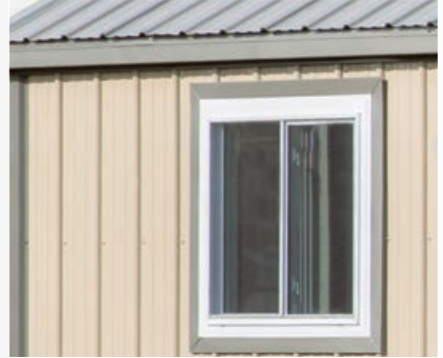
Metal Siding & Roofing
