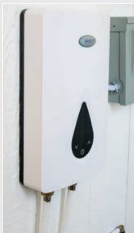
Electric Marey Tankless Water Heater 240 - V 60 AMP Circuit Domestic Water Supply Only
