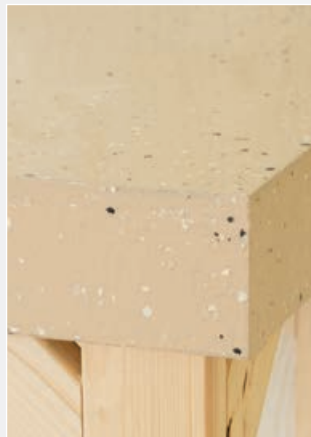
Detail of workshop w/Epoxy
