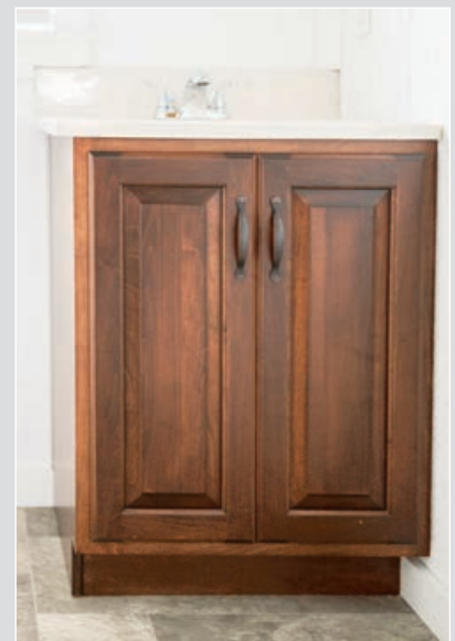
Vanity Cabinet - Installed
