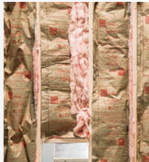
R-13 Batten Insulation In Walls & Ceiling
