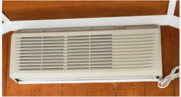
A/C Unit Installed
