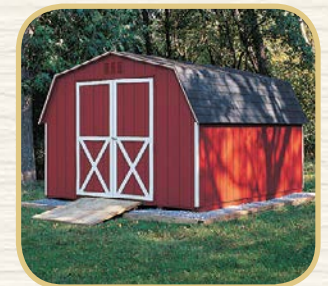
Stone Base Foundation
